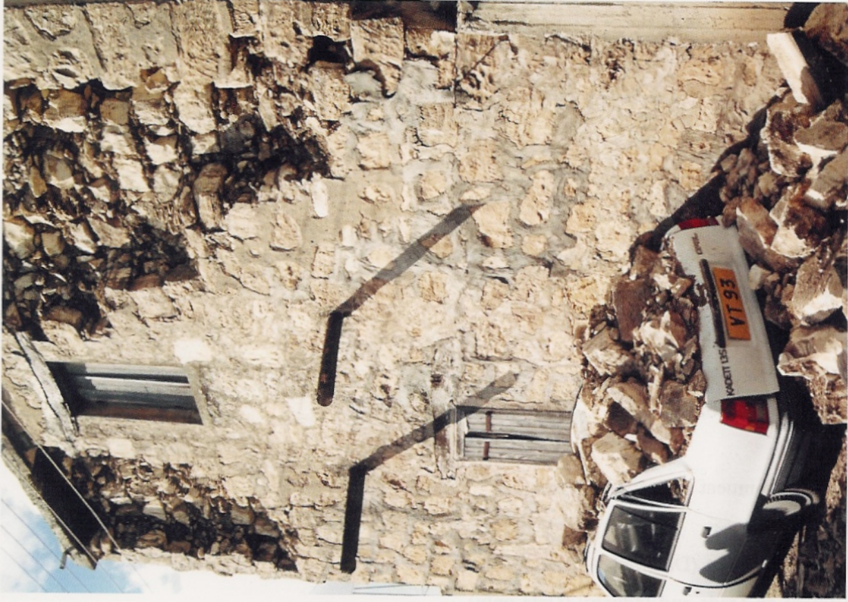
Plate 3. Damage caused by the magnitude 5.8 MB Cyprus earthquake of 23 February 1995 which caused the death of 2 people. (Photograph supplied by K Solomi, Cyprus Geological Survey).
