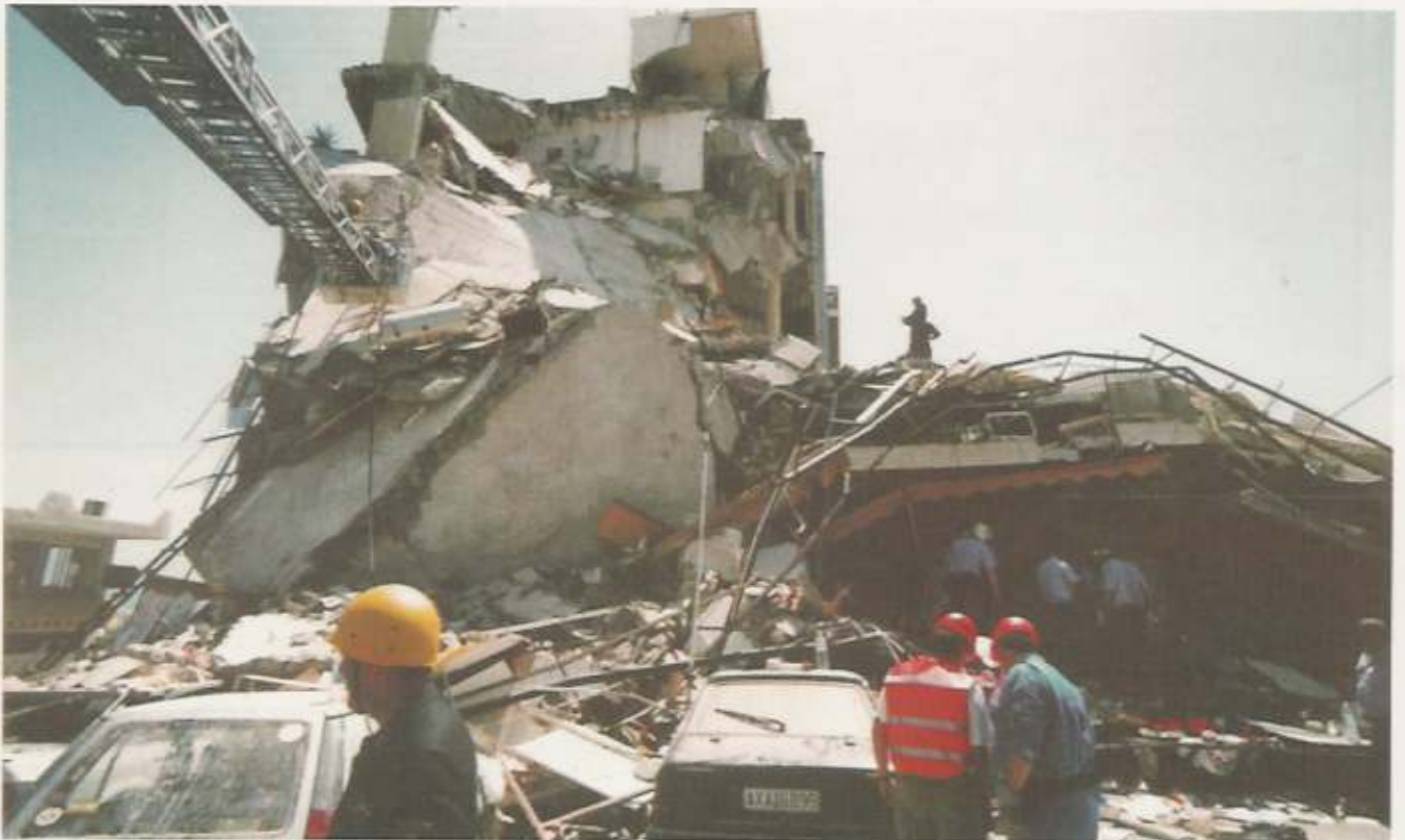
Plate 2. Damage caused by the magnitude 6.5 MS Greece earthquake of 15 June 1995 which resulted in the deaths of some 26 people. (Photograph supplied by Kathimerini, newspaper, Athens)
