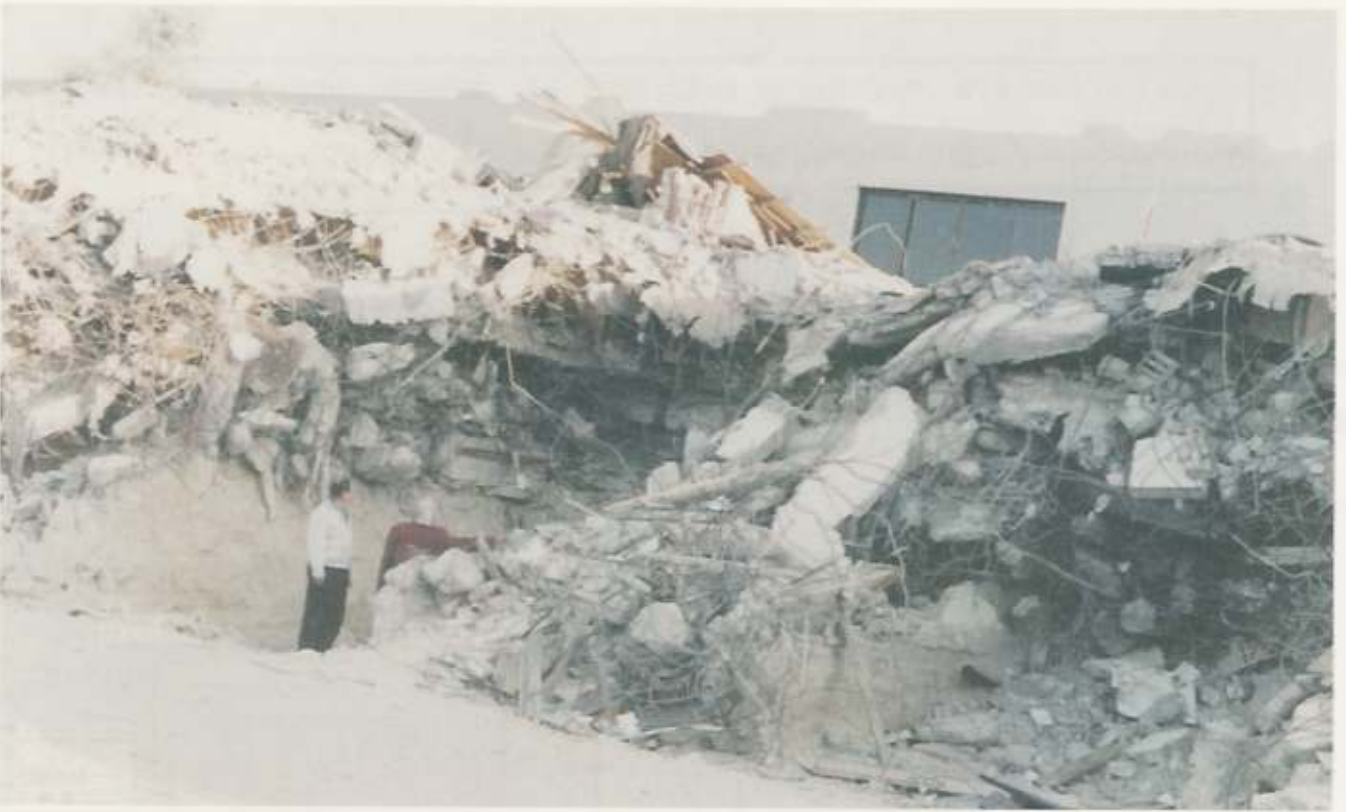
Plate 1. Damage caused by the magnitude 7.3 MS Gulf of Aqaba, Egypt earthquake of 22 November 1995 which caused the deaths of 8 people. (Photograph supplied by Amr Elnashi of Imperial College London)
